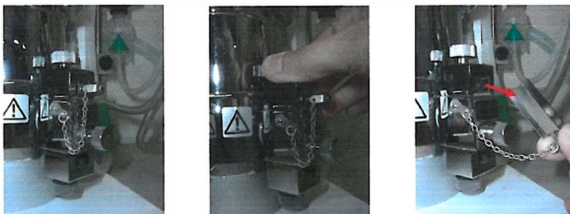
Figure 7: "Filling a Key-Fill Vaporizer"
